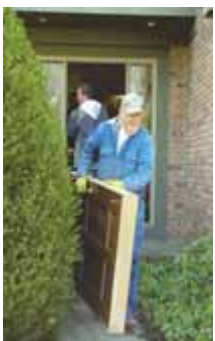
Volunteer Harold Ball removes a door from a recent deconstruction site.
